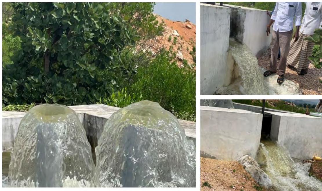
Figure 93: Lift Drop Point with left & right canals
